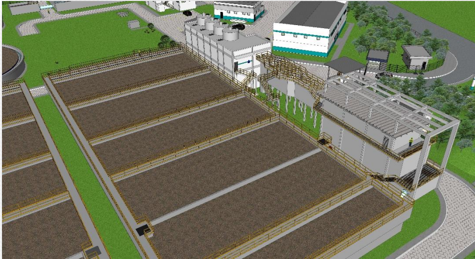
Tanque MBBR / Preliminar
