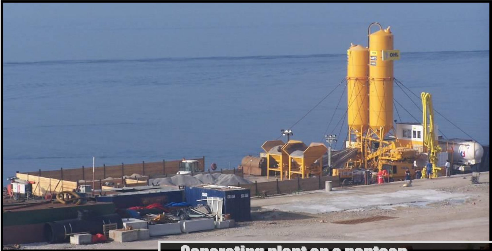
Concreting plant on a pontoon
